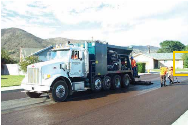
SLURRY SEAL
